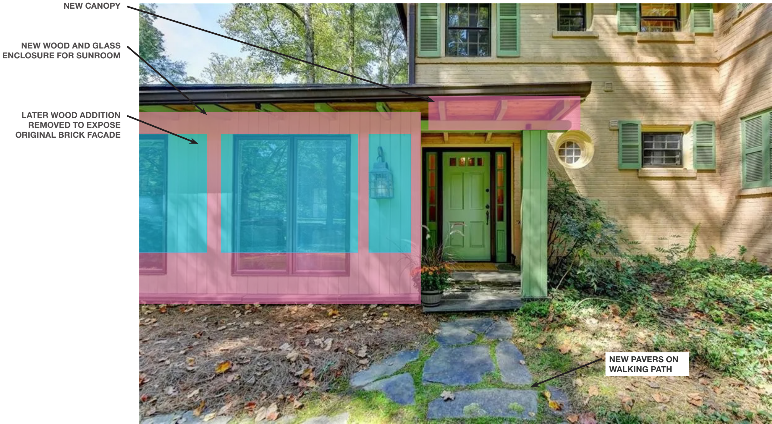
THIS IS AN ANACHRONISTIC ADDITION WHICH CLUTTERS UP THE ORIGINAL FACADE. WE WILL BE REBUILDING THIS AS A WOOD AND GLASS MORE OPEN ENCLOSURE THAT CONCEALS LESS OF THE HISTORIC BUILDING.
