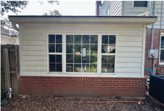
Rear Façade with Knee Wall and Hardie Plank Siding
