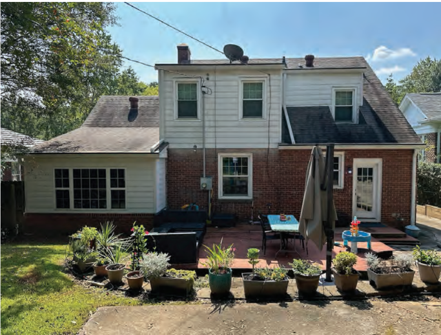
Rear Façade (North Elevation)
