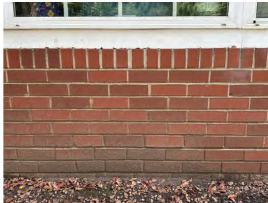
Close-up of Bricks on Knee Wall on Rear Façade
