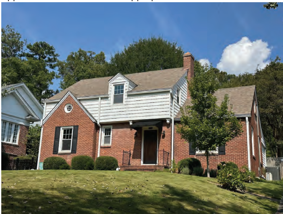
South and East Elevations
