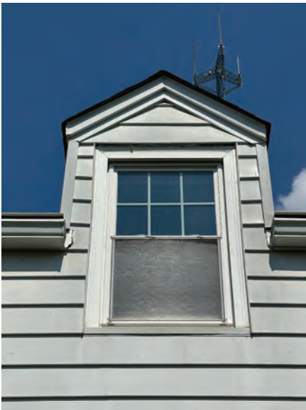
Six-Over-One Window on Front Façade to Match
