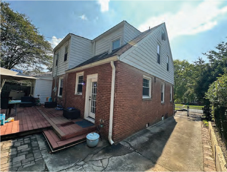
West Elevation Seen from Rear of House
