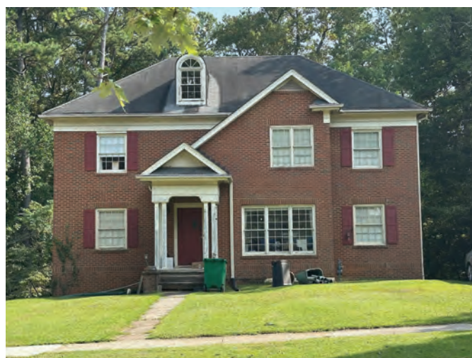
1369 Emory Road NE
