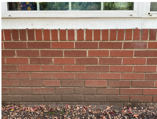
Close-up of Bricks on Knee Wall on Rear Façade
