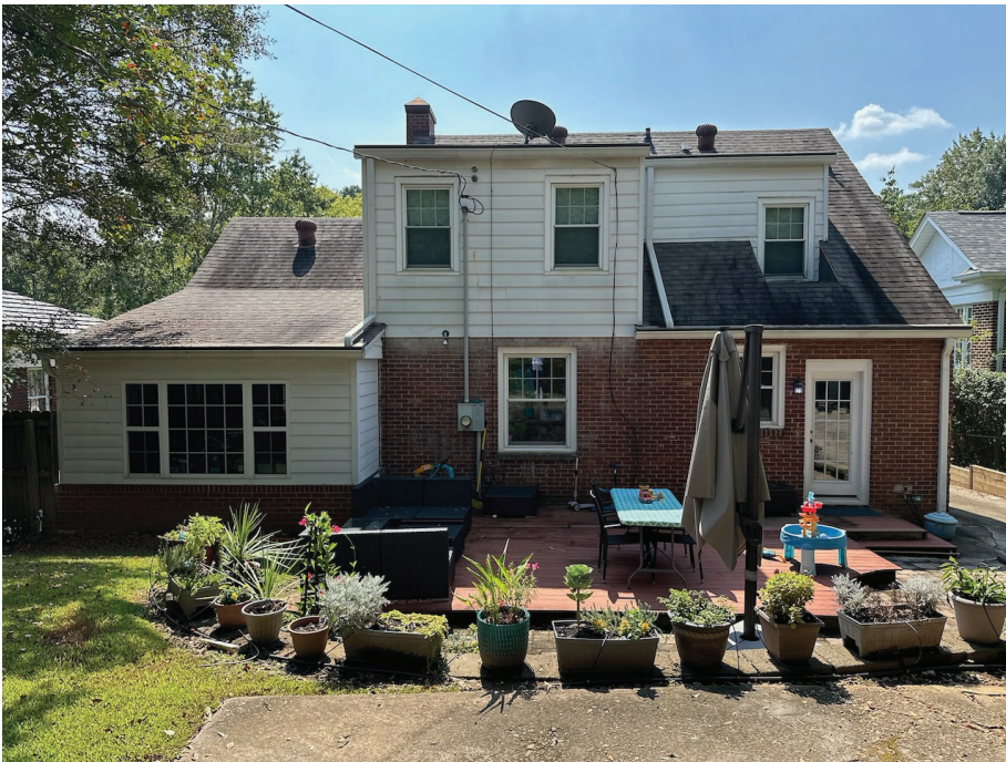
Rear Façade (North Elevation)
