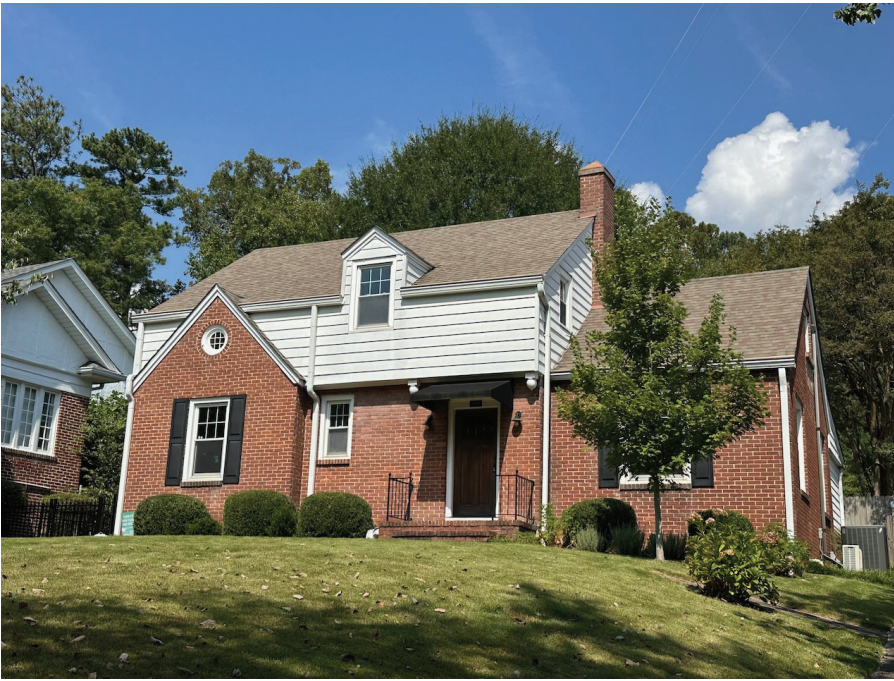
South and East Elevations
