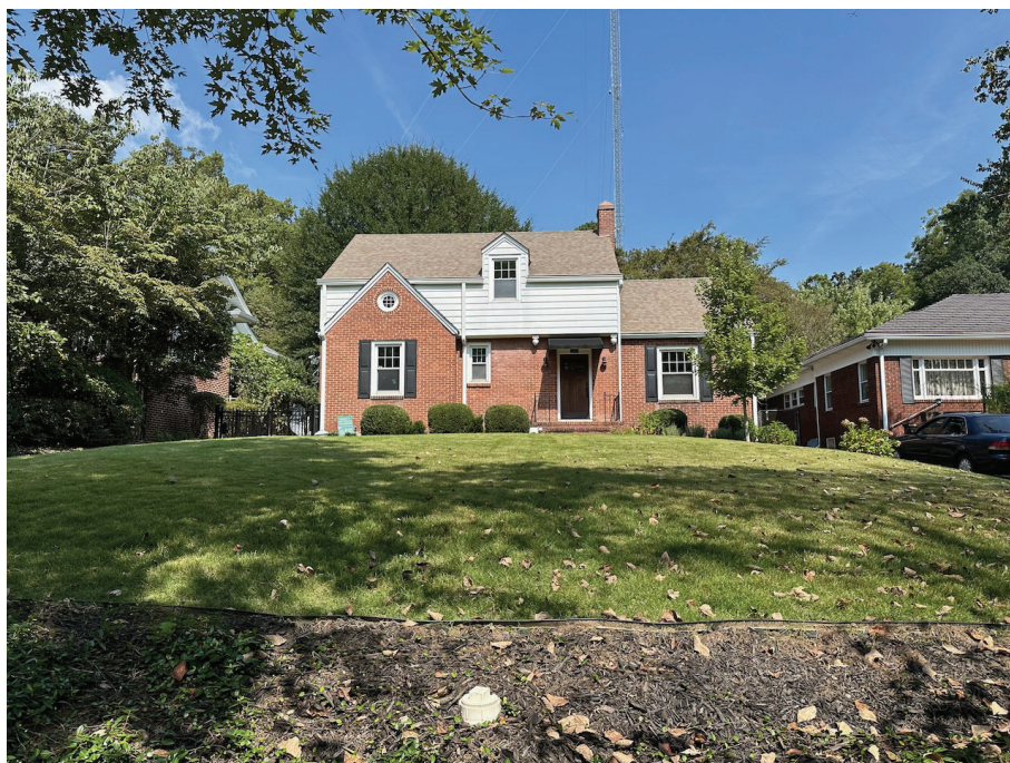
Front Façade (South Elevation) Showing Adjacent Houses
