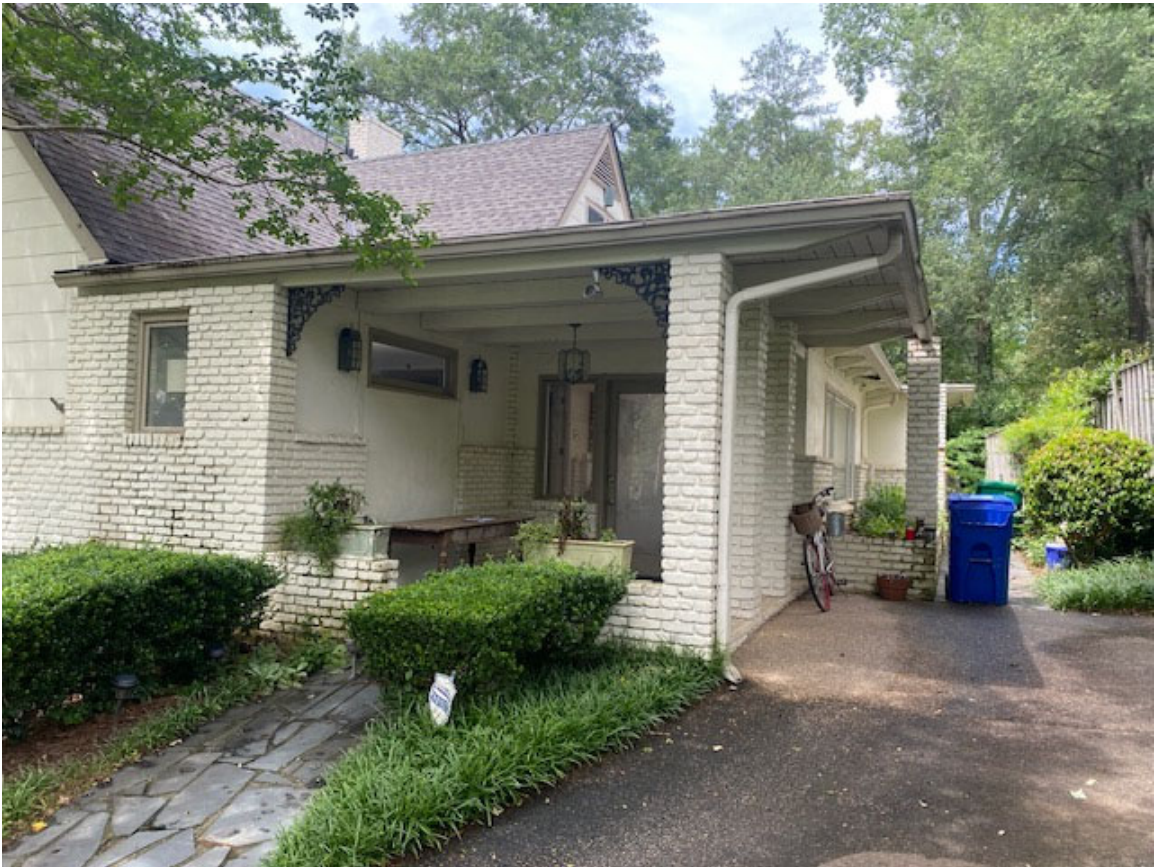
View of the Enclosed Carport and Covered Entry
