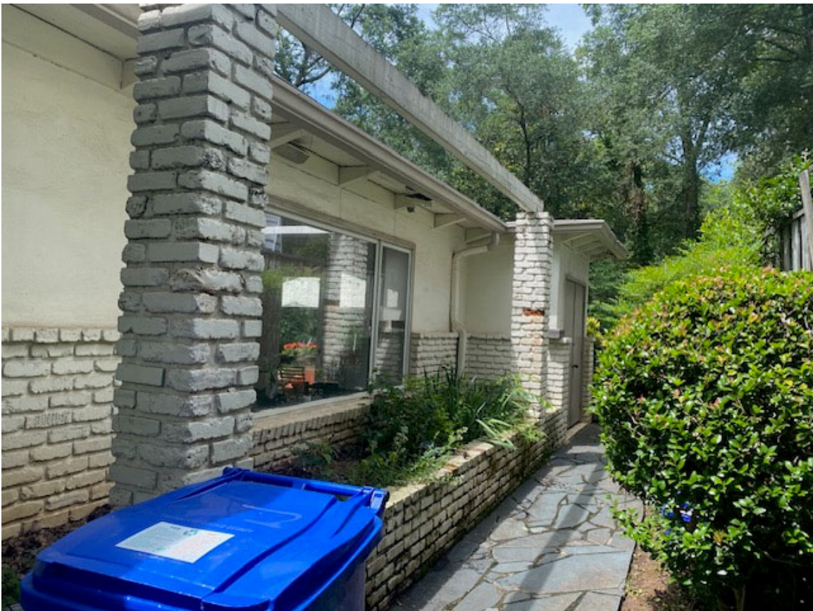
View Along the Right Side of the House
