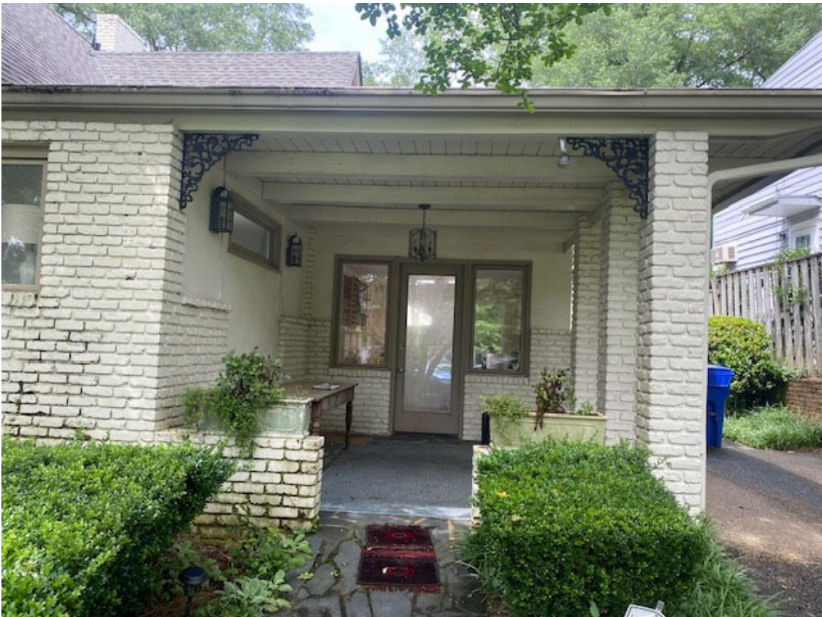
View of Entry
