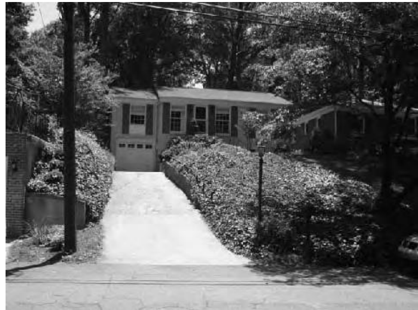
Example of integral front-loading garage, Coventry Drive.
