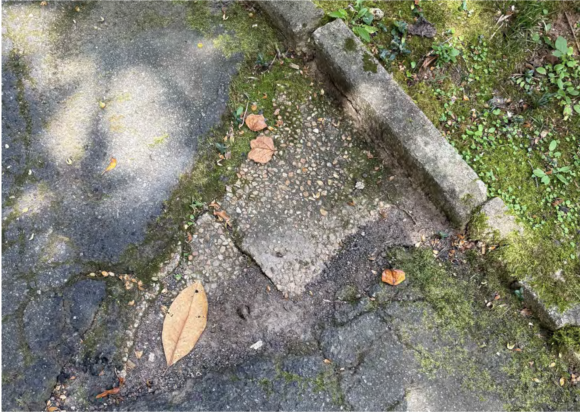
EXISTING EXPOSED AGGREGATE DRIVEWAY UNDER ASPHALT
