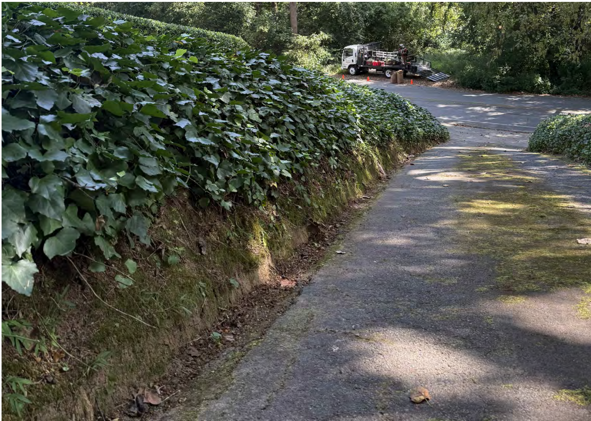
ERODED SLOPE ALONG DRIVEWAY
