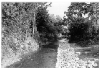
View of Lullwater Creek illustrating the use of "gabions." Gabions are large, fenced cages filled with rock, placed along the bankside to arrest erosion.
