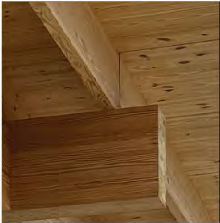
SOUTHERN YELLOW PINE RAFTERS & ROOF SOFFIT CLADDING
