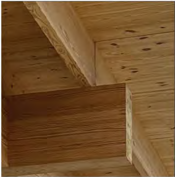
SOUTHERN YELLOW PINE RAFTERS & ROOF SOFFIT CLADDING
