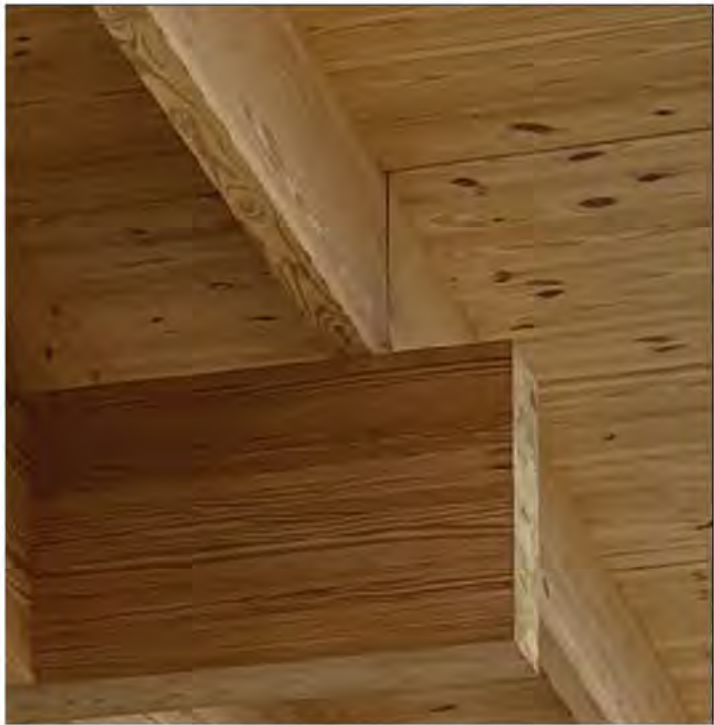
SOUTHERN YELLOW PINE RAFTERS & ROOF SOFFIT CLADDING
