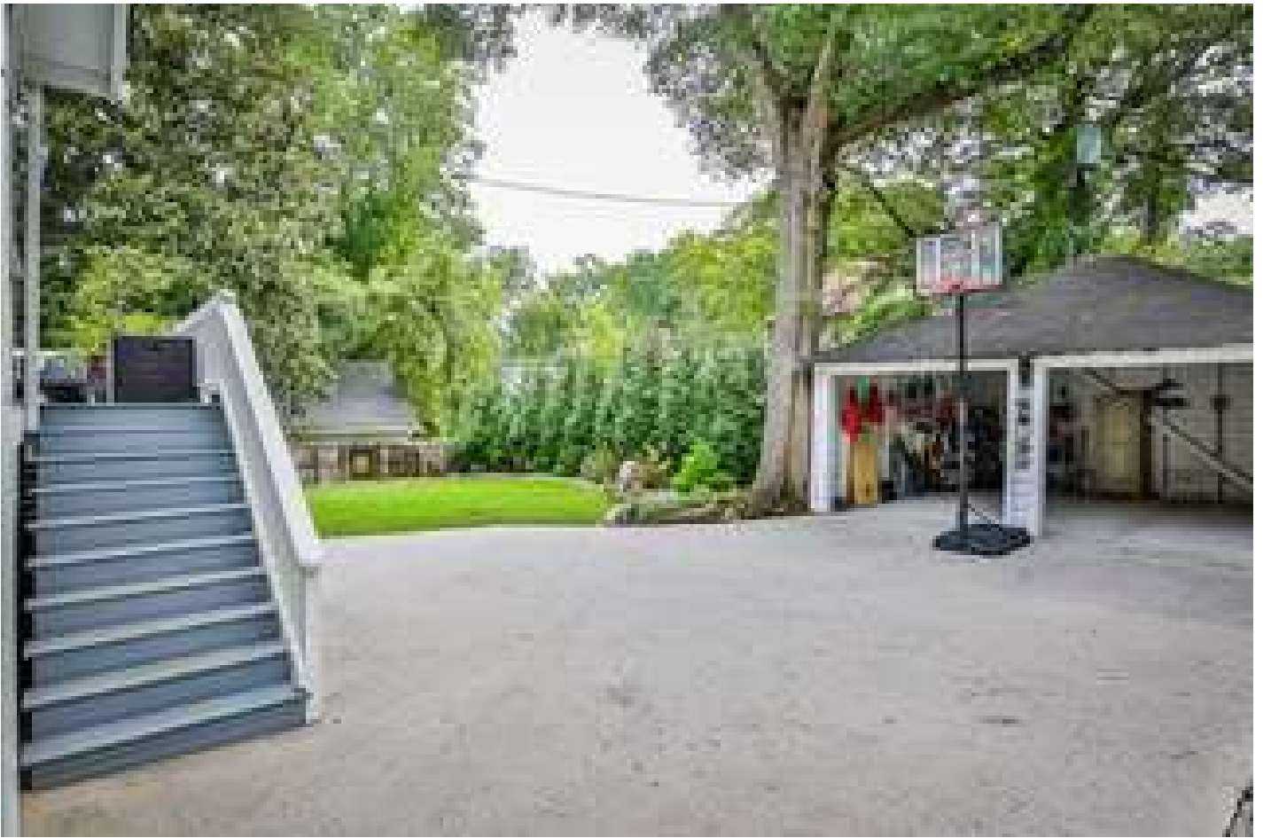
Photo of recently demolished garage – note lack of any braced portal framing and exterior siding attached directly to studs with no structural sheathing. Stud spacing is more than two feet on center and were rotten where they were in contact with the concrete slab. The concrete slab foundation, driveway, and minimal turnaround are existing and will remain.
