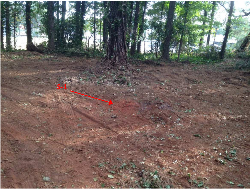
Completed Borehole and Surrounding Area, Boring Location S-1
