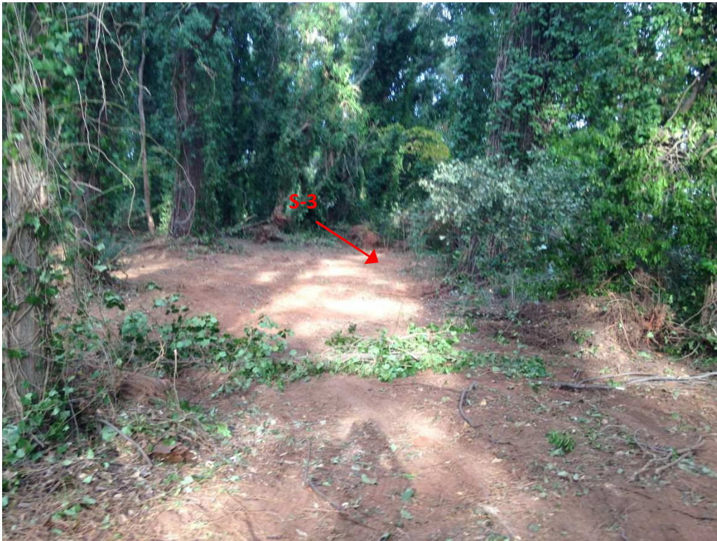
Completed Borehole and Surrounding Area, Boring Location S-3
