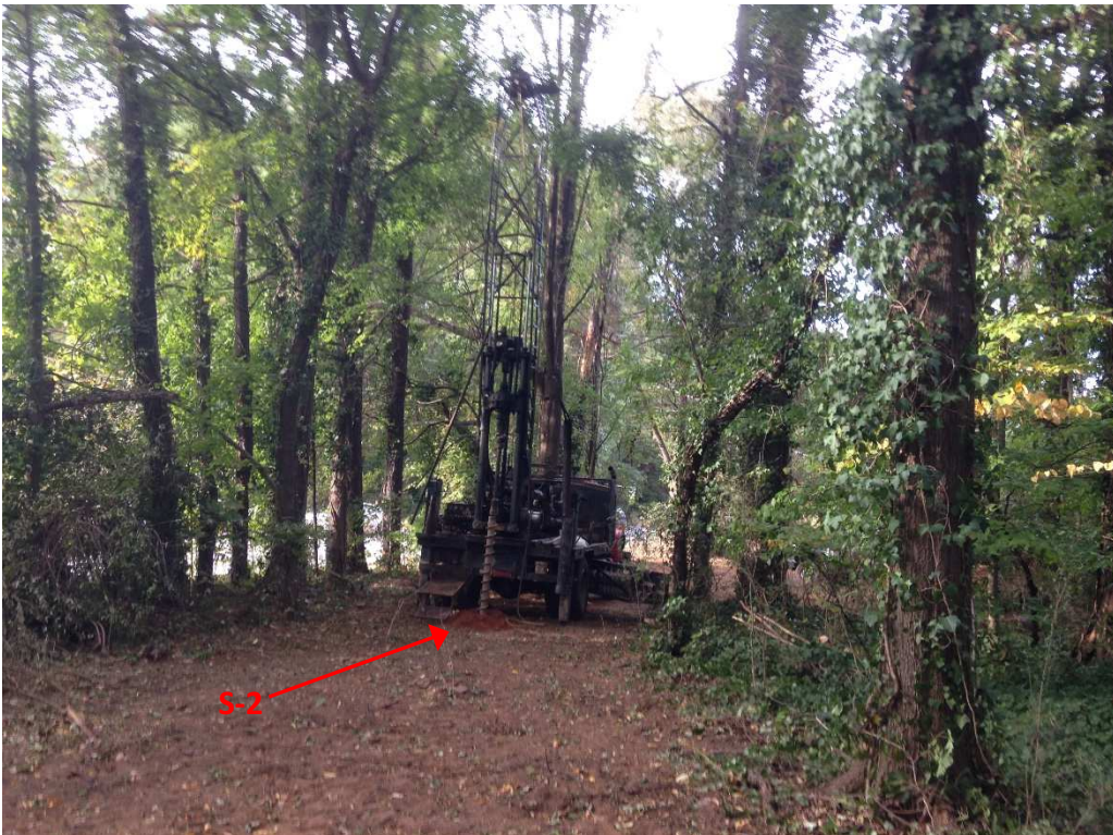
Drill Rig Set-up, Boring Location S-2
