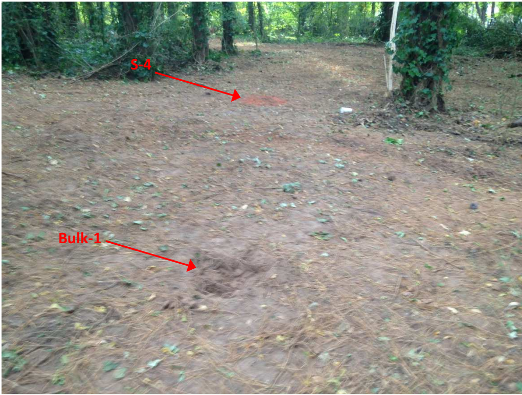
Completed Borehole and Surrounding Area, Boring Locations S-4 and Bulk-1
