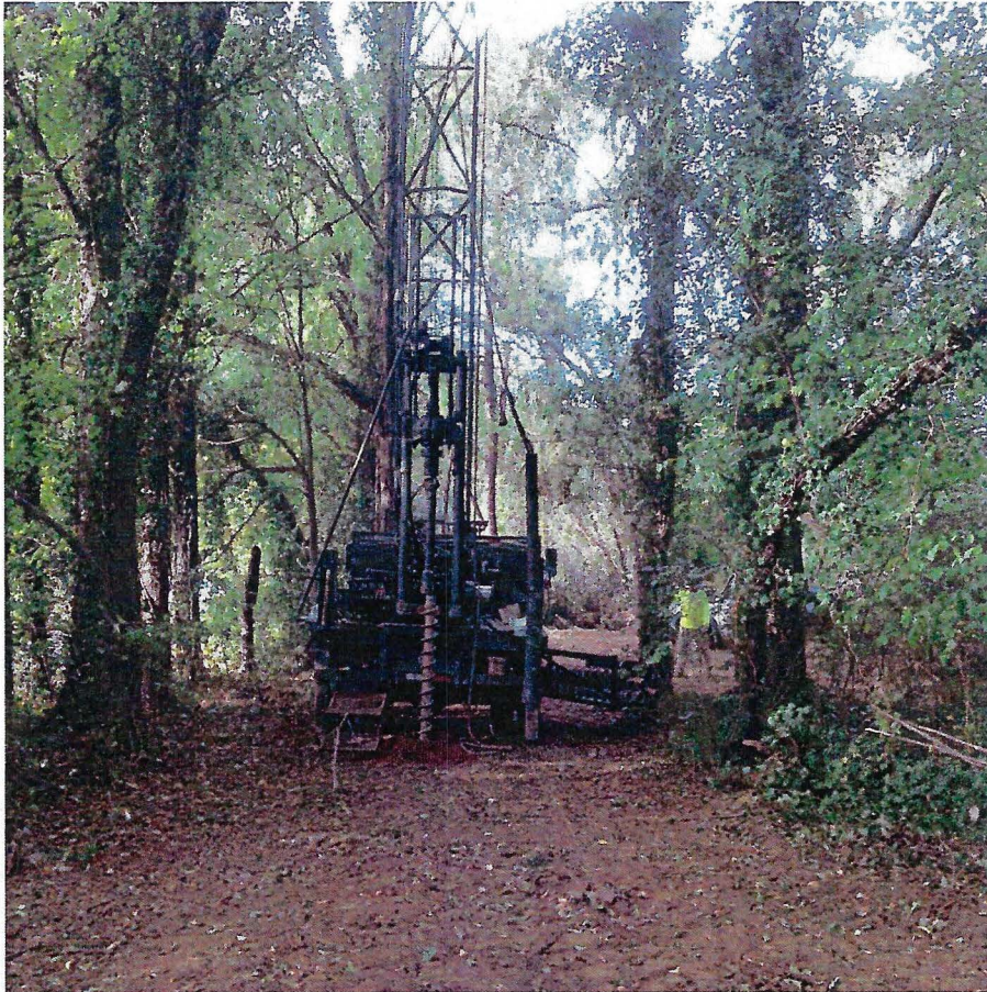
Drill Rig Set-up, Location S-2
