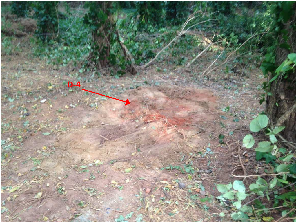
Completed Borehole and Surrounding Area, Boring Location D-4
