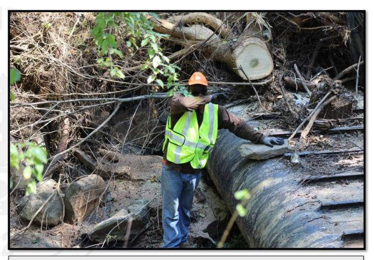
On Aug. 23, 2017, a record 6.4 million gallons of sewage spilled into Snapfinger Creek. The spill was caused by a 16-inch-diameter tree growing out of a concrete junction box.
