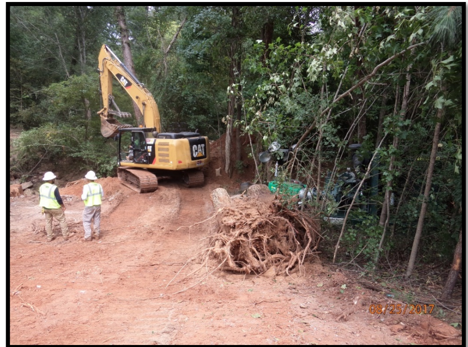
DeKalb County crews work to remove a large tree that caused the Snapfinger Creek spill in August 2017.
