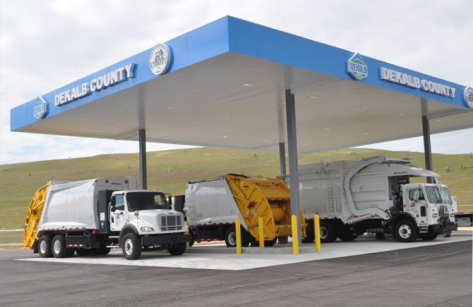
CNG Station – Seminole Road Landfill
