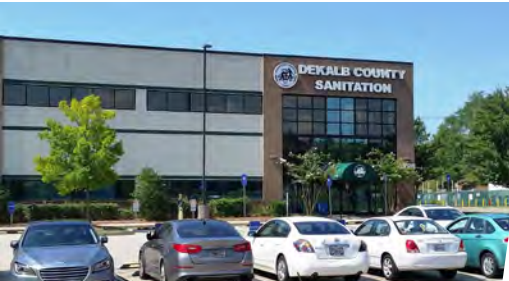
Sanitation Division administrative office
