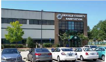
Sanitation Division Administrative Office
