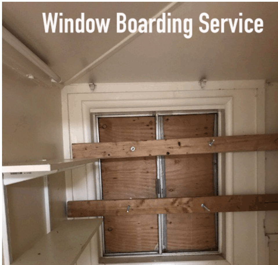
Picture 2 – Boarding up sliding windows
