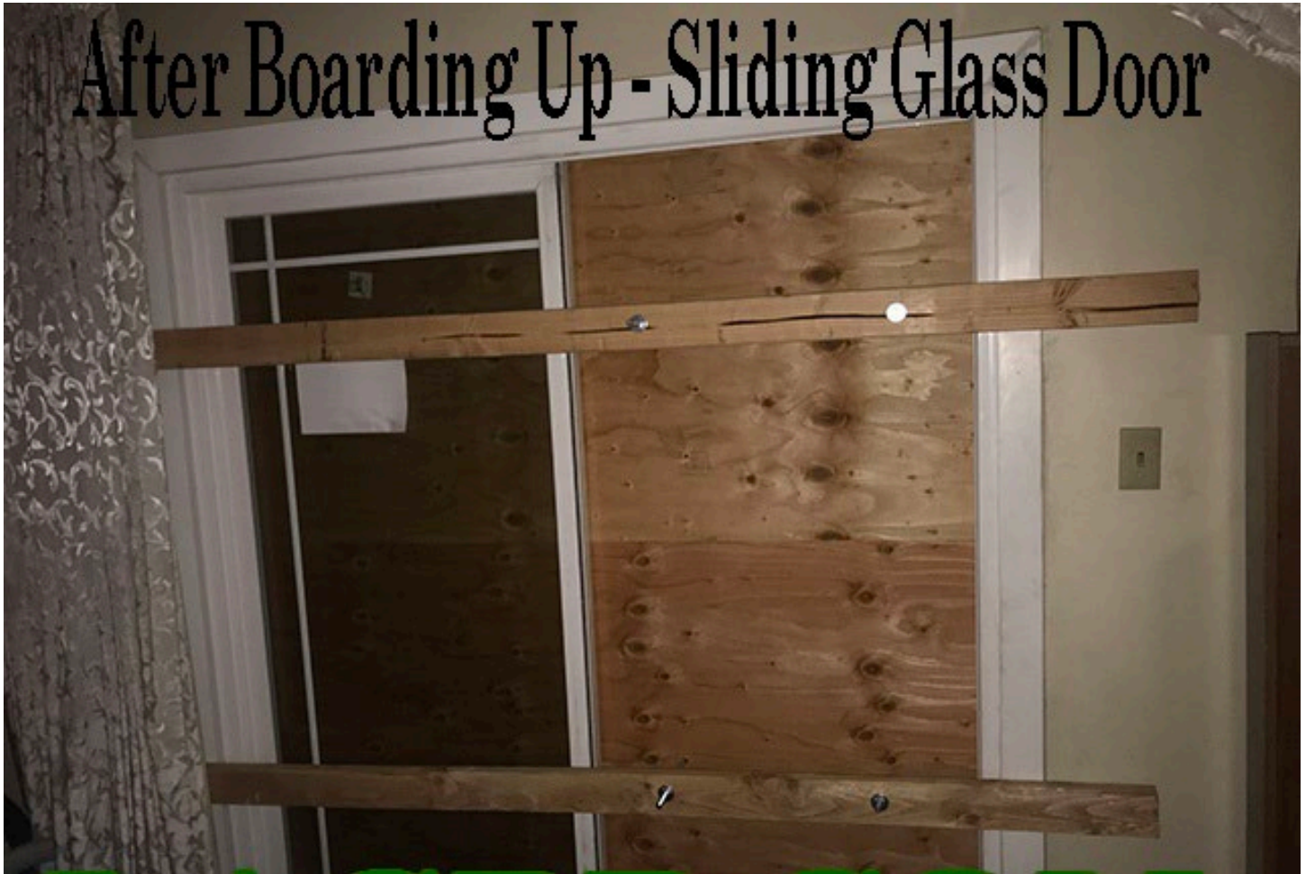
Picture 1 – Boarding up sliding glass doors
