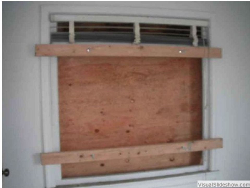
Picture 3 – Boarding up sliding windows
