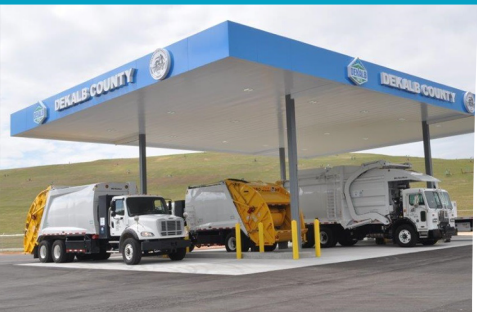
CNG Station – Seminole Road Landfill
