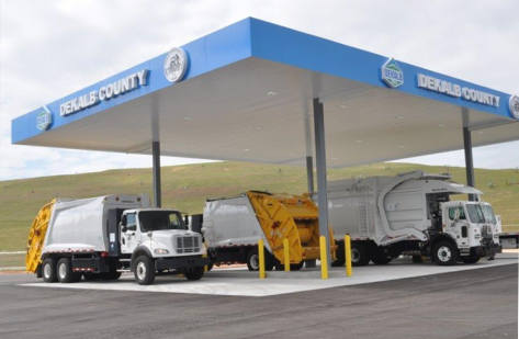
CNG Station – Seminole Road Landfill
