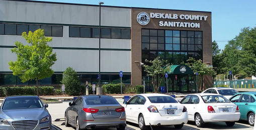
Sanitation Division Administrative Office
