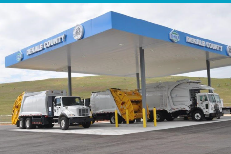
CNG Station – Seminole Road Landfill
