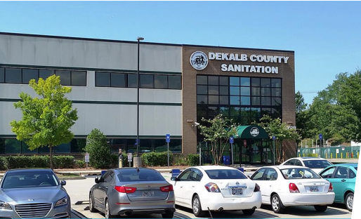
Sanitation Division Administrative Office
