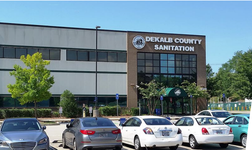
Sanitation Division Administrative Office
