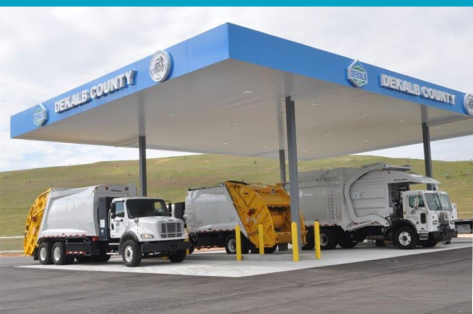
CNG Station – Seminole Road Landfill
