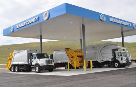
CNG Station – Seminole Road Landfill
