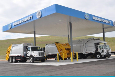
CNG Station – Seminole Road Landfill
