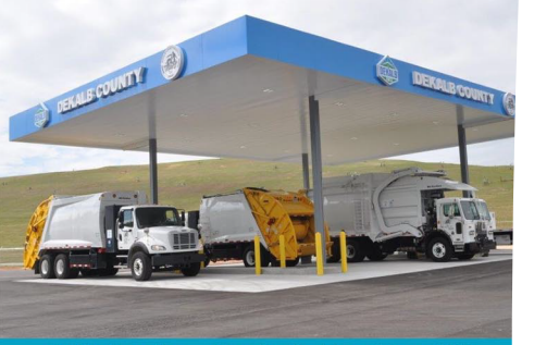
CNG Station – Seminole Road Landfill
