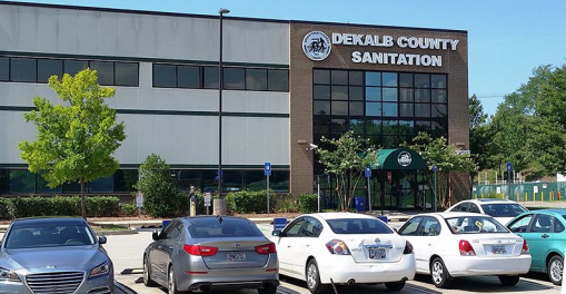
Sanitation Division Administrative Office
