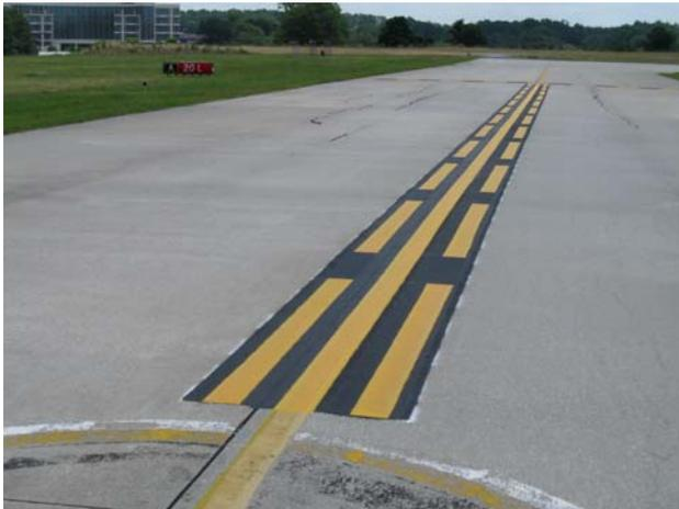
Of additional interest, Instrument Landing System (ILS) hold short marking and lighting has been installed on Taxiway ‘A’ and Taxiway ‘J’ approaching Runway 20 Left. Technically, these markings and signs control the Precision Object Free Zone (POFZ) for the Runway 20Left ILS. The POFZ is a volume of airspace that must be kept clear when an aircraft is on a vertically guided final approach (ILS). The POFZ becomes “active” when the reported weather at PDK is
