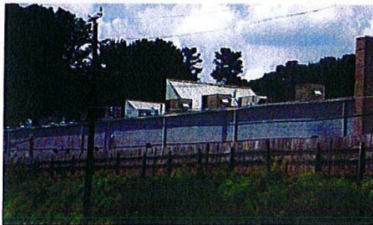
This is not adequate screening or detailing
