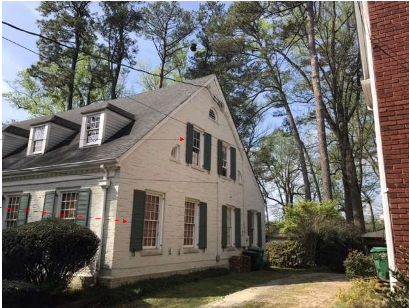
1096 Clifton Road – Driveway Side Opposite side elevation matches
