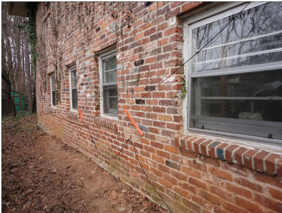
AS BUILT CONDITIONS WEST
