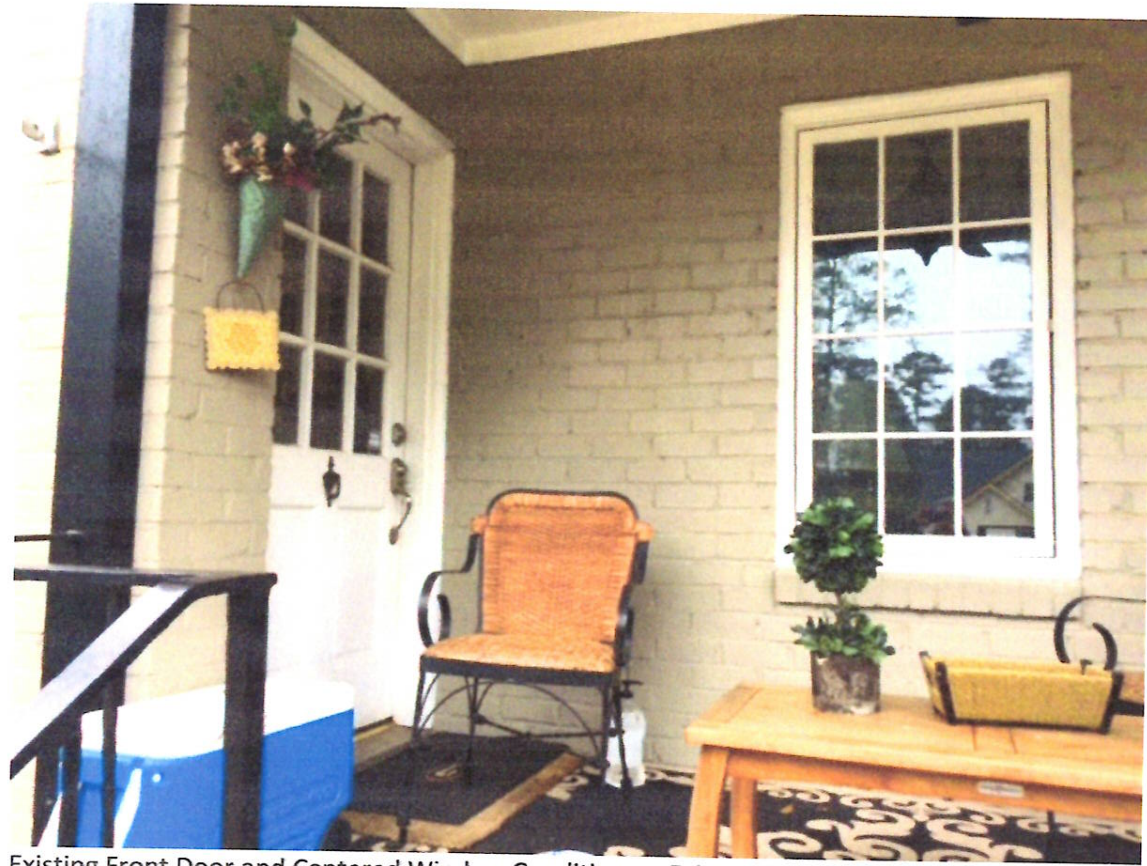
Existing Front Door and Centered Window Condition on Existing Entry Porch
