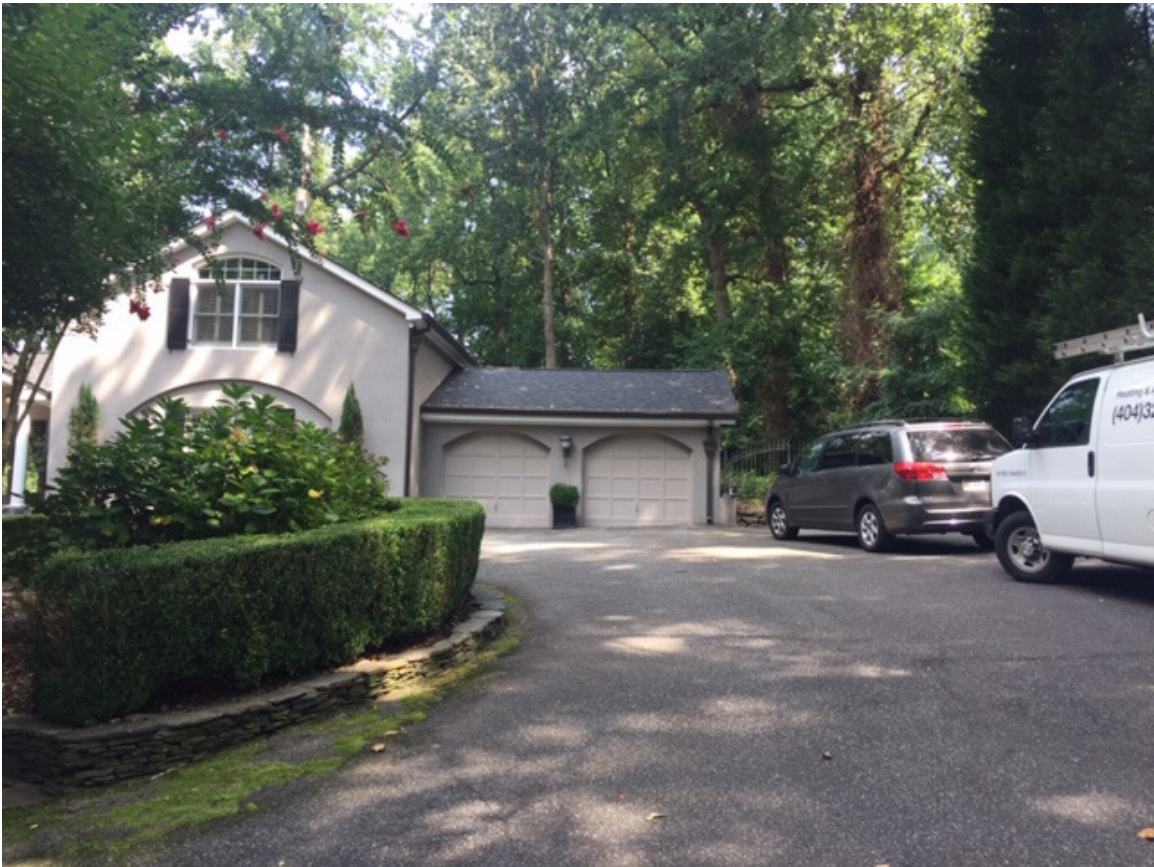
View of Attached Garage
