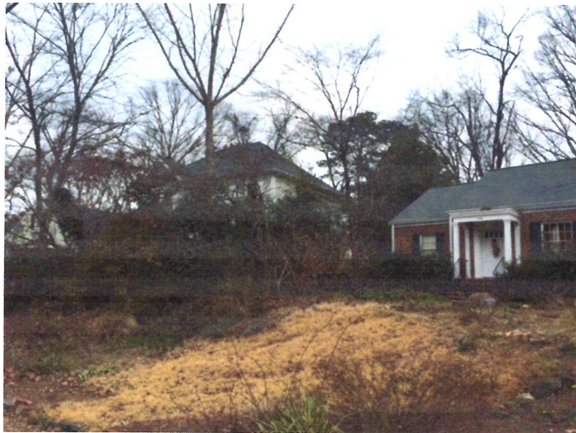
View from Right-of-Way Along East Façade (Proposed porch and dining room window addition)
