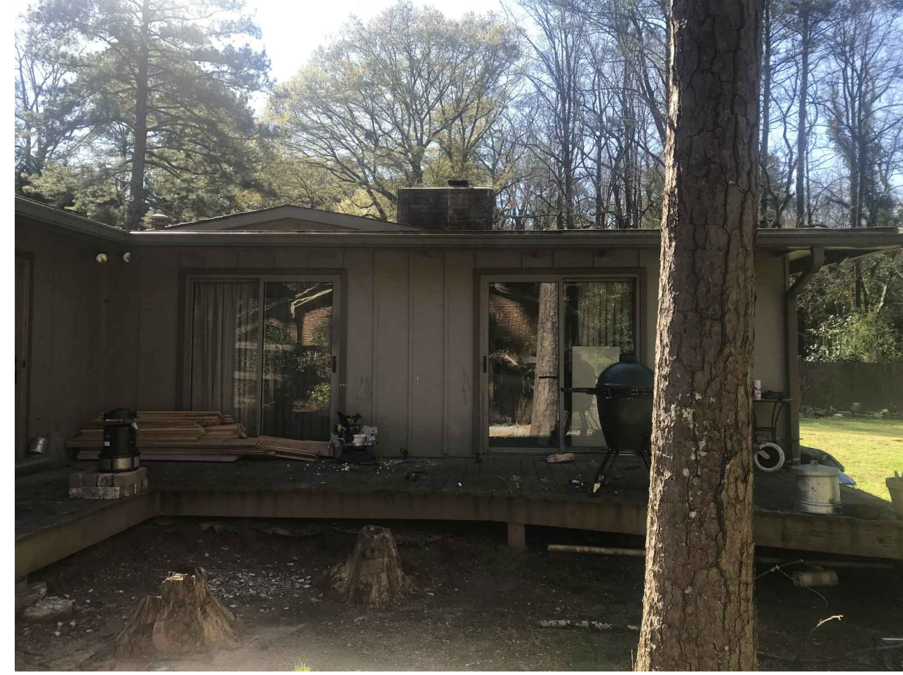
EXISTING NORTH FACADE
