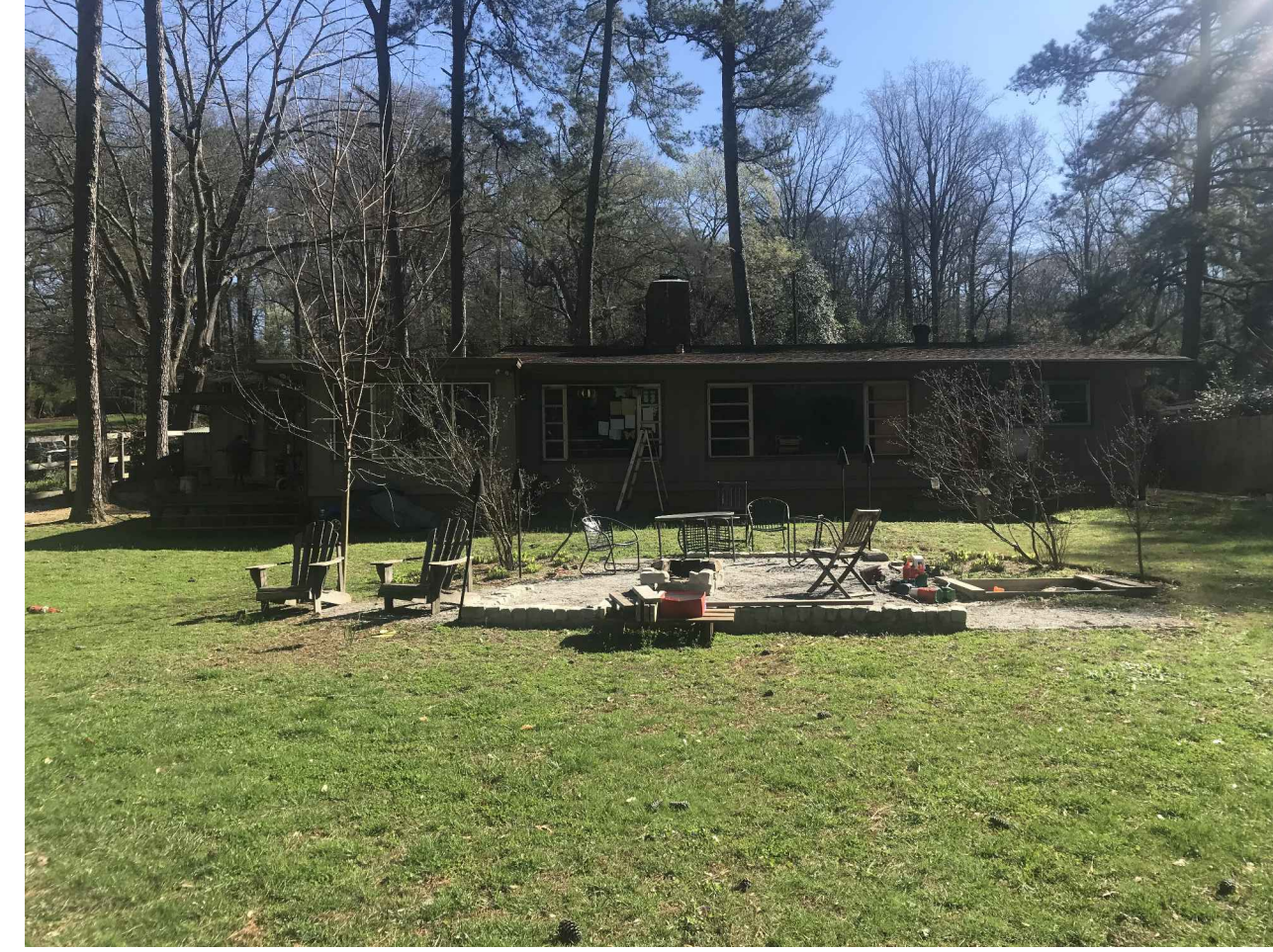
EXISTING REAR FACADE
