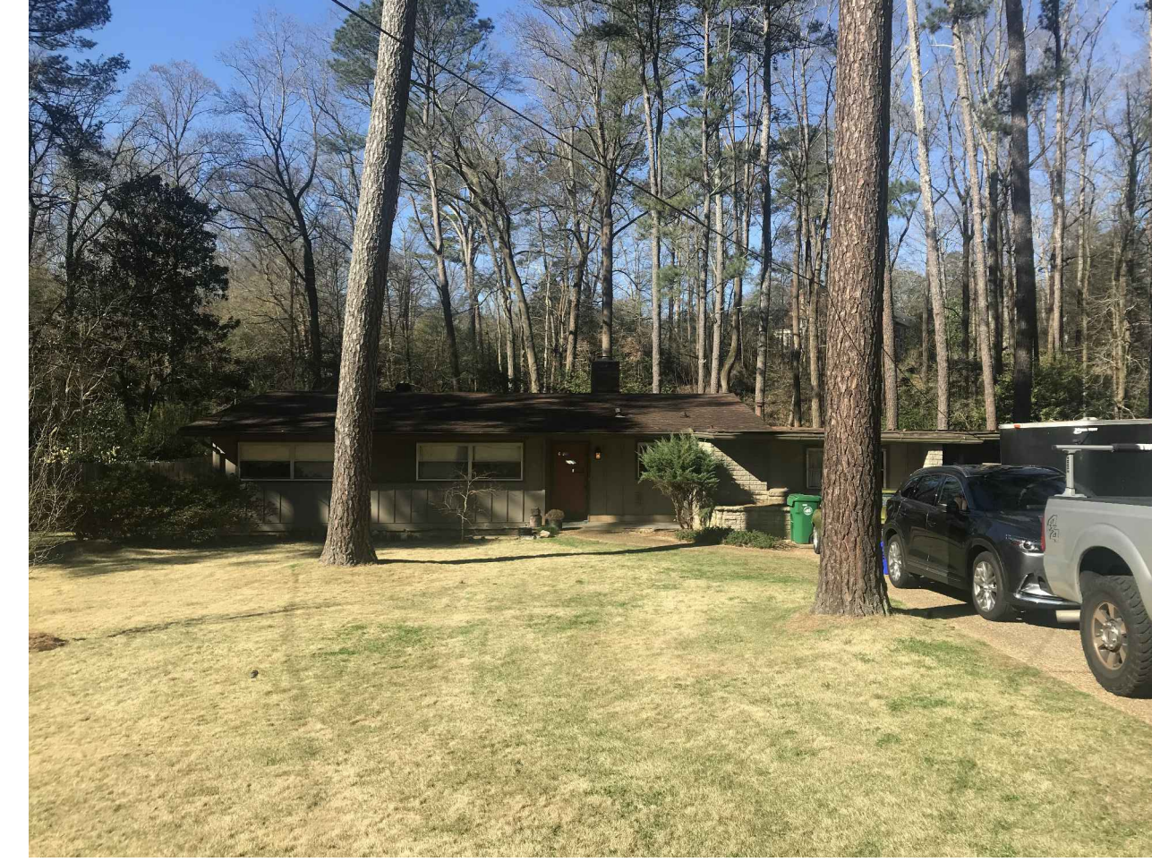
EXISTING FRONT FACADE
