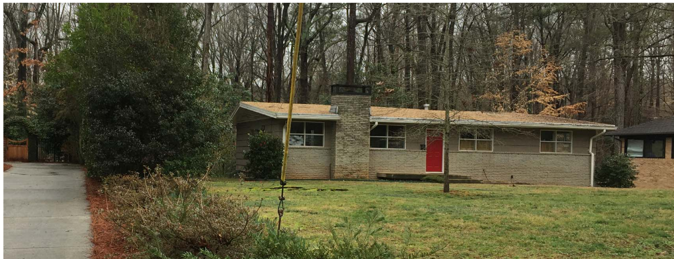
WEST ELEVATION, FROM RIGHT OF WAY / 894 BARTON WOODS ROAD NE ATLANTA, GA 30307
