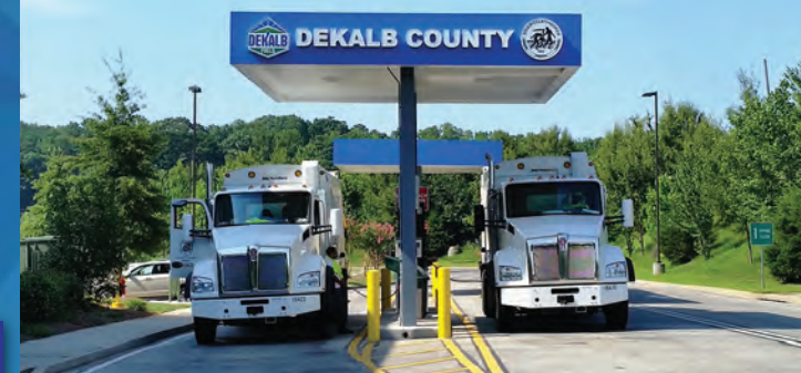
Sanitation Division Public CNG Fueling Station
