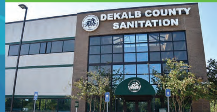
Sanitation Division Administration Building
