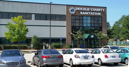
Sanitation Division Administrative Office
