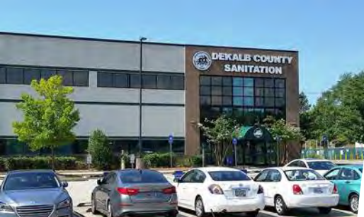
Sanitation Division Administrative Office
