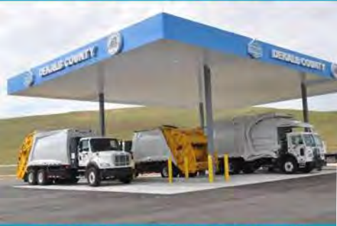
CNG Station - Seminole Road Landfill
