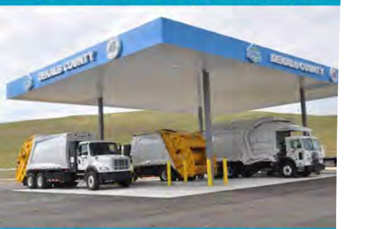
CNG Station - Seminole Road Landfill
