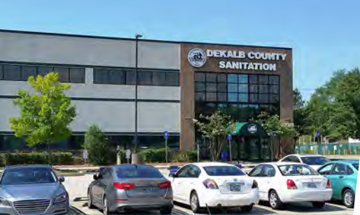
Sanitation Division Administrative Office
