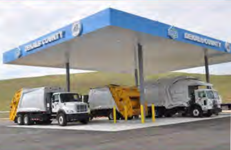
CNG Station - Seminole Road Landfill
