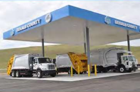
CNG Station – Seminole Road Landfill
