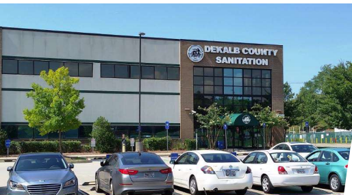
Sanitation Division Administrative Office
