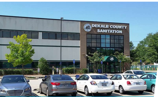
Sanitation Division Administrative Office
