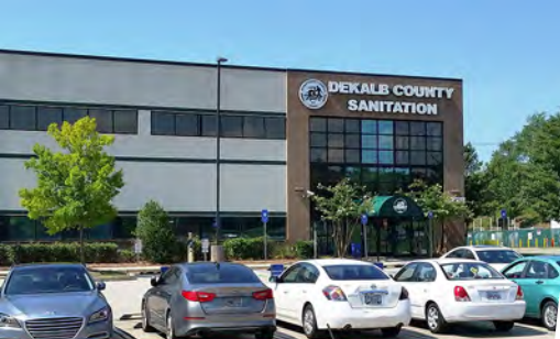
Sanitation Division Administrative Office
