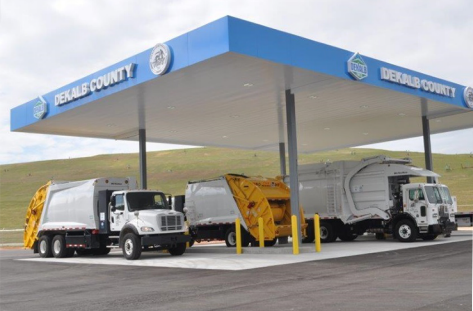
CNG Station – Seminole Road Landfill
