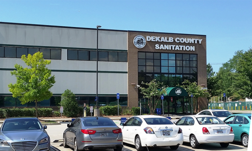
Sanitation Division Administrative Office
