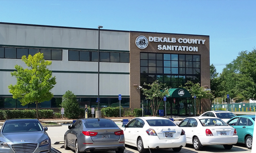
Sanitation Division Administrative Office
