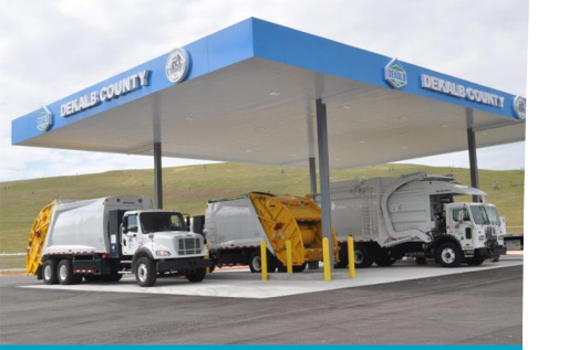
CNG Station – Seminole Road Landfill
