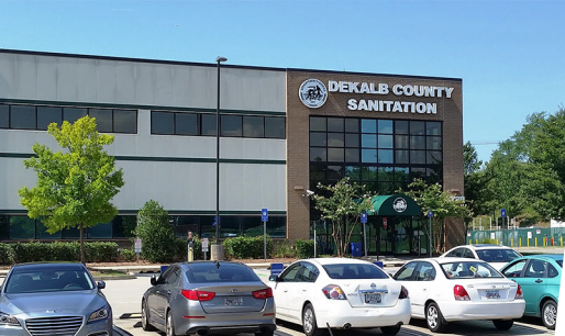
Sanitation Division Administrative Office
