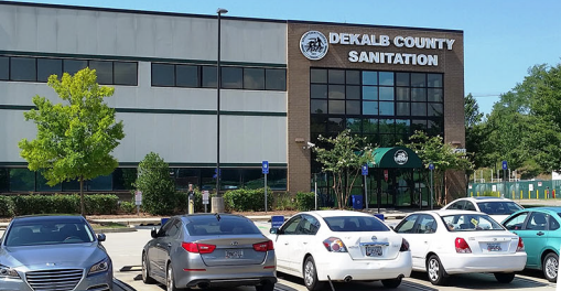
Sanitation Division Administrative Office
