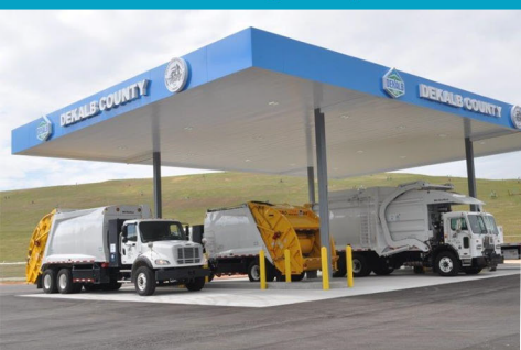
CNG Station – Seminole Road Landfill
