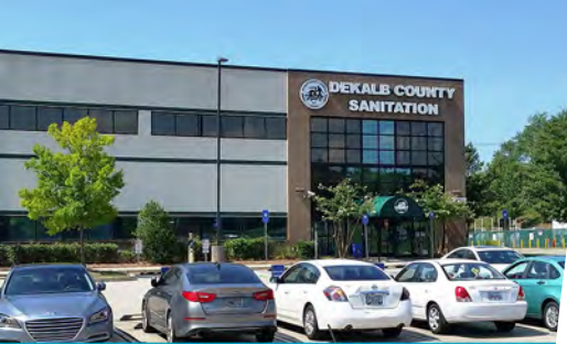
Sanitation Division Administrative Office
