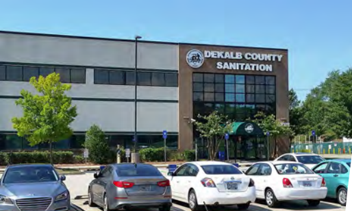
Sanitation Division Administrative Office
