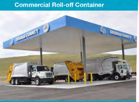
CNG Station – Seminole Road Landfill
