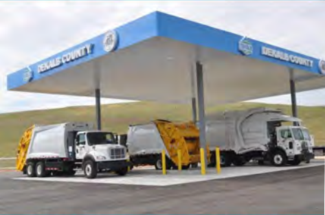
CNG Station – Seminole Road Landfill
