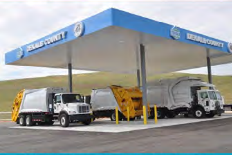
CNG Station – Seminole Road Landfill
