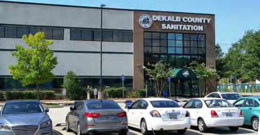
Sanitation Division Administrative Office
