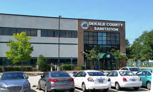
Sanitation Division Administrative Office
