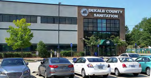
Sanitation Division Administrative Office
