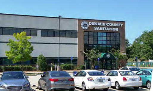
Sanitation Division Administrative Office
