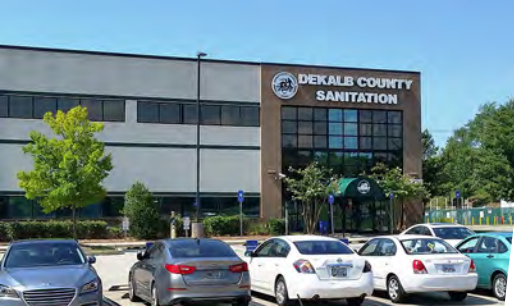
Sanitation Division Administrative Office
